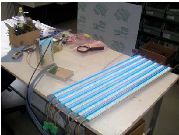
controller, power supply and LED-stripes in the test
